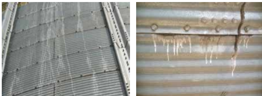
Figure 1: Formation of white strips outside of silos as a result of moisture condensation.
